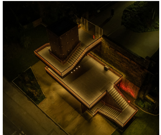
Wellington Place, Viaduct Link - Leeds
